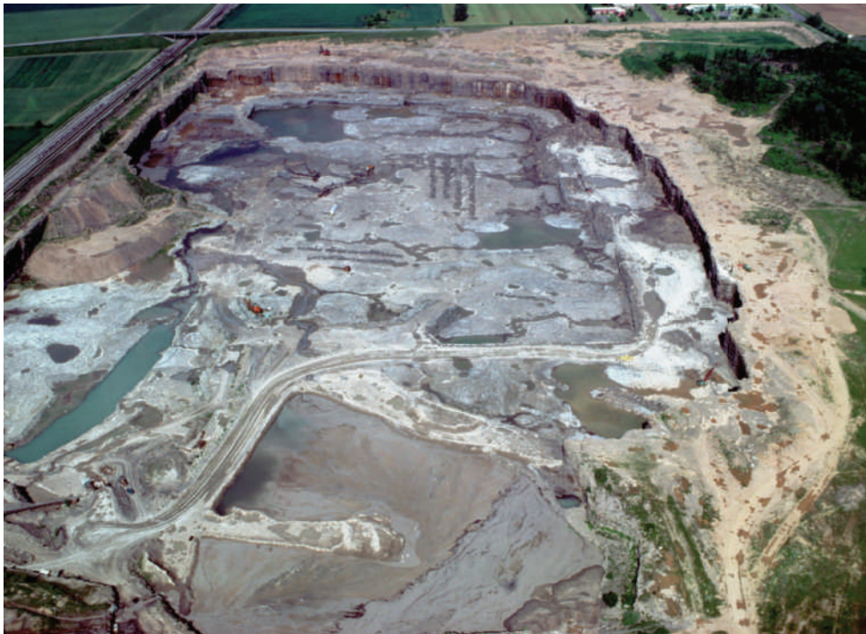
Figure 21-22 Surface impoundment in Niagara Falls, New York (USA). Such sites can pollute the air and nearby groundwater and surface water.
