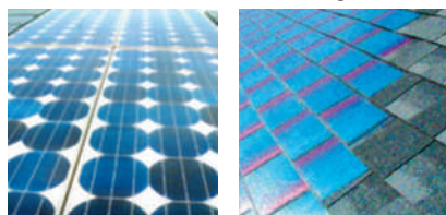
Figure 16-17 Solutions: Photovoltaic (PV) or solar cells can provide electricity for a house or other building using solar-cell roof shingles, as shown in this house in Richmond Surrey, England. Solar-cell roof systems that look like a metal roof are also available. In addition, new thin-film solar cells can be applied to windows and outside walls.
