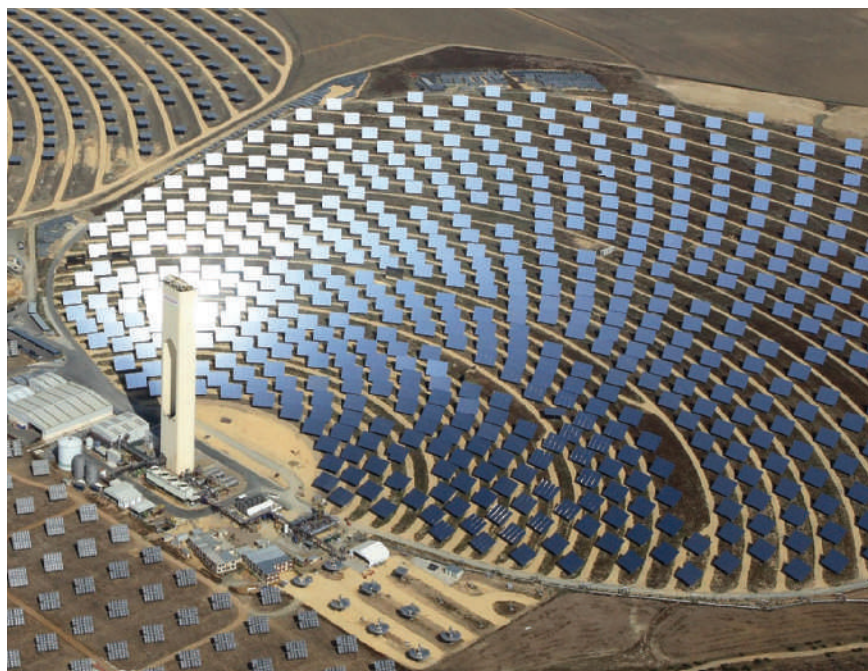
Figure 16-15 Solutions: Commercial solar power tower plant operated by Solúcar, an Abengoa company, near the city of Seville in southern Spain. This plant, which began operating in 2007, uses an array of 624 mirrors to reflect and focus sunlight on a receiver atop a 35-story tower. The resulting concentrated heat converts water into steam that spins turbines and generates enough electricity to power 6,000 homes.
