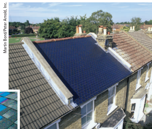
Figure 16-17 Solutions: Photovoltaic (PV) or solar cells can provide electricity for a house or other building using solar-cell roof shingles, as shown in this house in Richmond Surrey, England. Solar-cell roof systems that look like a metal roof are also available. In addition, new thin-film solar cells can be applied to windows and outside walls.
