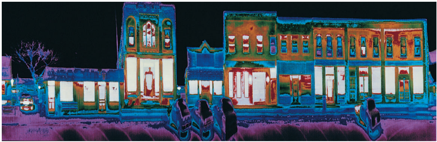
Figure 16-8 A thermogram , or infrared photo, showing heat loss (red, white, and orange) around the windows, doors, roofs, and foundations of houses and stores in Plymouth, Michigan. Many homes and buildings in the United States and other countries are so full of leaks that their heat loss in cold weather and heat gain in hot weather are equivalent to what would be lost through a large window-sized hole in a wall of the house. Question: How do you think the place where you live would compare to these houses in terms of heat loss?
