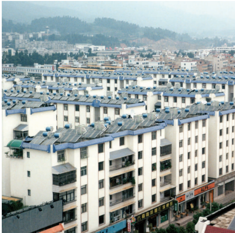
Figure 16-12 Rooftop solar hot water heaters on apartment buildings in the Chinese city of Kunming in the Yunnan province. Such heaters are now required on all new buildings and their use is growing rapidly in urban and rural areas of China.
