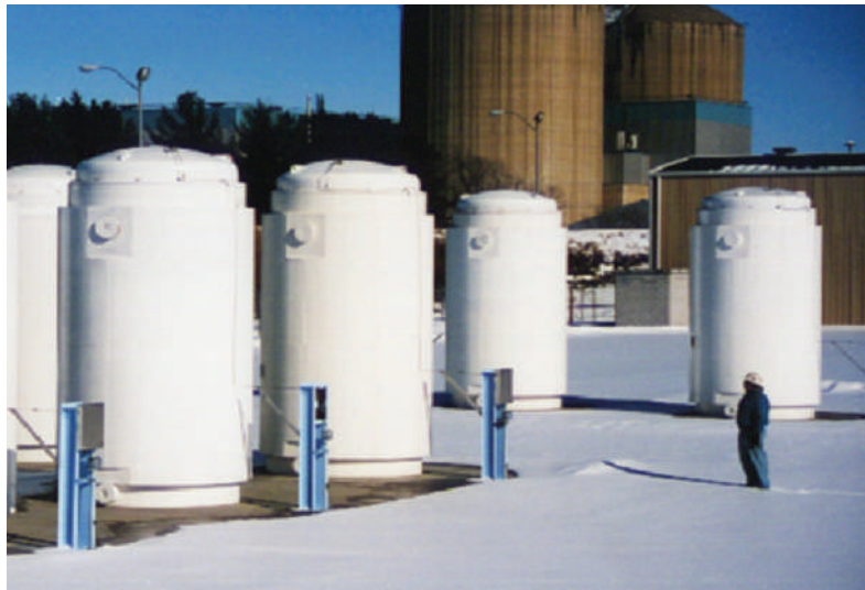
Figure 15-18 Science: after 3 or 4 years in a reactor, spent fuel rods are removed and stored in a deep pool of water contained in a steel-lined concrete basin (left). After they have cooled considerably, some fuel rods are stored upright on concrete pads (right) in dry-storage containers made of steel or concrete. Question: Do you think these are safe storage methods? Why or why not?
