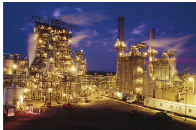
Figure 15-4 Science: refining crude oil. Components of petroleum are removed at various levels, depending on their boiling points, in a giant distillation column. The most volatile components with the lowest boiling points are removed at the top of the column. The photo shows an oil refinery in the U.S. state of Texas.
